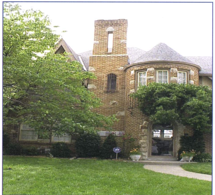
An exterior chimney will often make it more difficult to start a fire.
