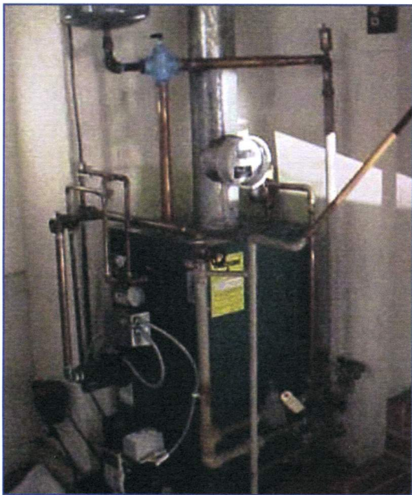
By allowing dilution air to enter the venting system downstream of the appliance, a barometric draft regulator reduces draft.
