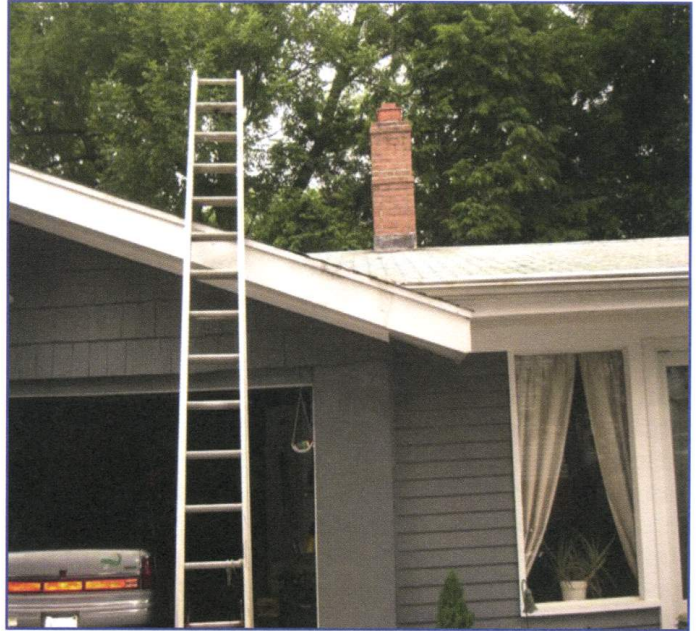
An interior chimney works better than one exposed to the outside.
